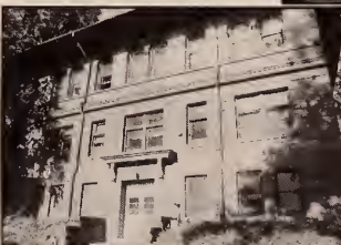
Weaver Building on the University park Campus
